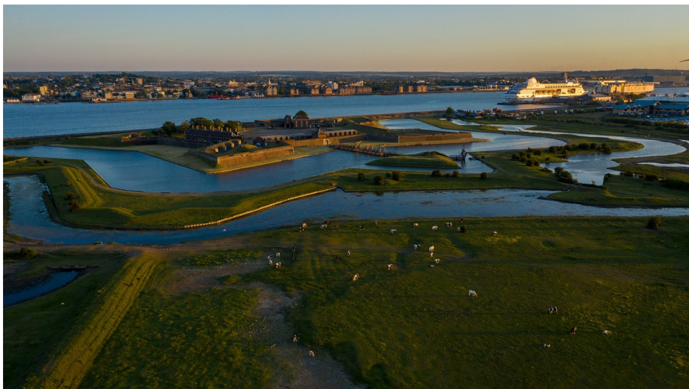
Tilbury Fort and London International Cruise Terminal, Port of Tilbury
